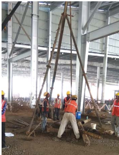
Fig. 2. Borehole in progress inside the factory structure
