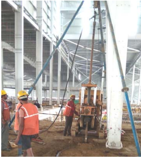
Fig. 14. Coring through pile in progress
