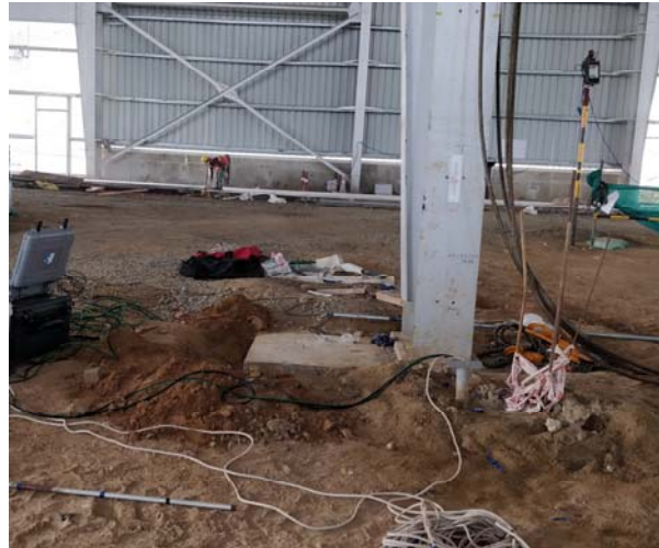
Fig. 11. Borehole for parallel seismic test adjacent to pile cap
