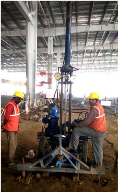
Fig. 3. Static cone penetration test in progress
