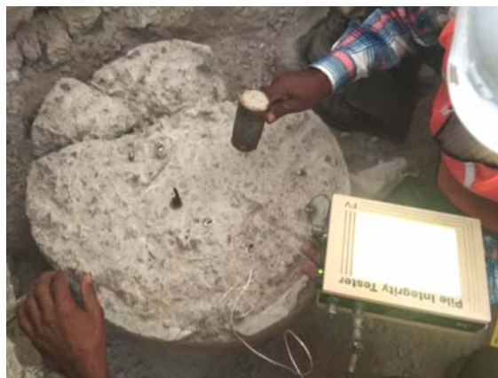
Fig. 5. Pile integrity test in progress
